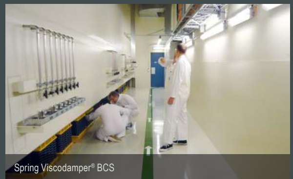
Spent Fuel Storage Tank with BCS – NPP Gösgen, Switzerland
